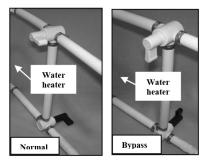
Two Valve Water Heater Bypass
